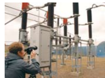
Gas detection from safe distance
